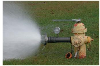
Figure 4-6. A Hydrant Being Flowed with a Diffuser as Part of a Fire-Flow Test.
